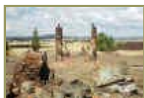
Close-up view of wooden support legs.
