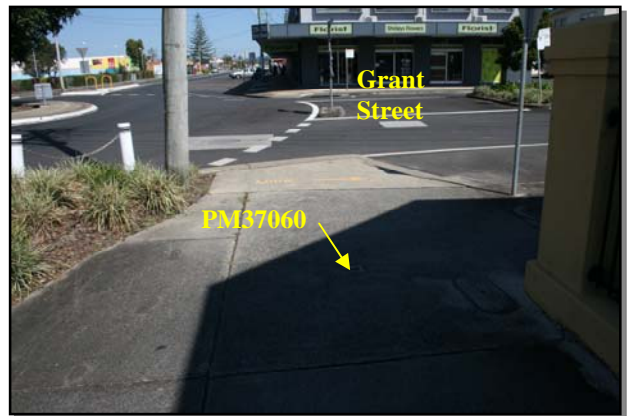
Figure 6.9 – PM37060 Intersection on 24/10/10
