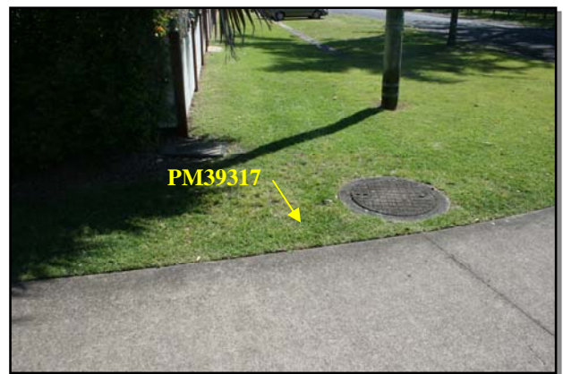
Figure 6.6 – PM39317 Intersection on 24/10/10
