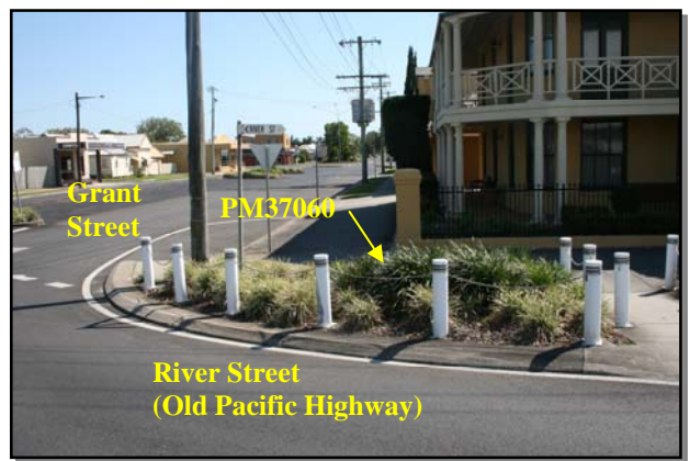
Figure 6.8 – PM37060 Intersection on 24/10/10
