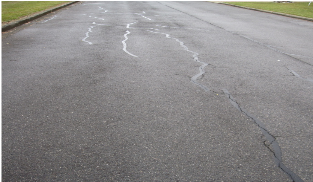
Figure 3.14 – Longitudinal cracking photo
