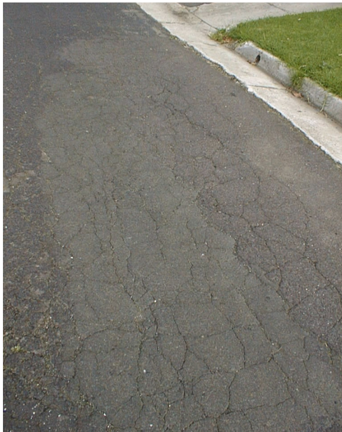
Figure 3.11 – Crocodile cracking photo
