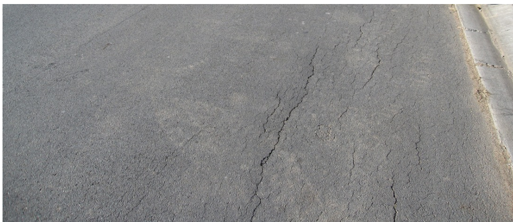
Figure 6.2 – Photo of Site 020 showing longitudinal cracking subsequent to subgrade deformation
