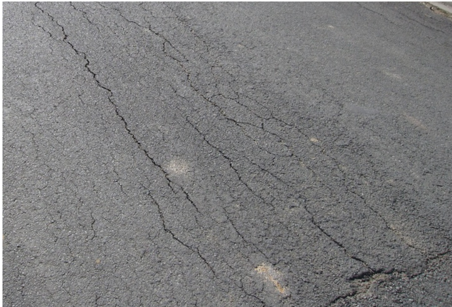
Figure 6.1 – Photo of Site 018 showing longitudinal cracking subsequent to subgrade deformation
