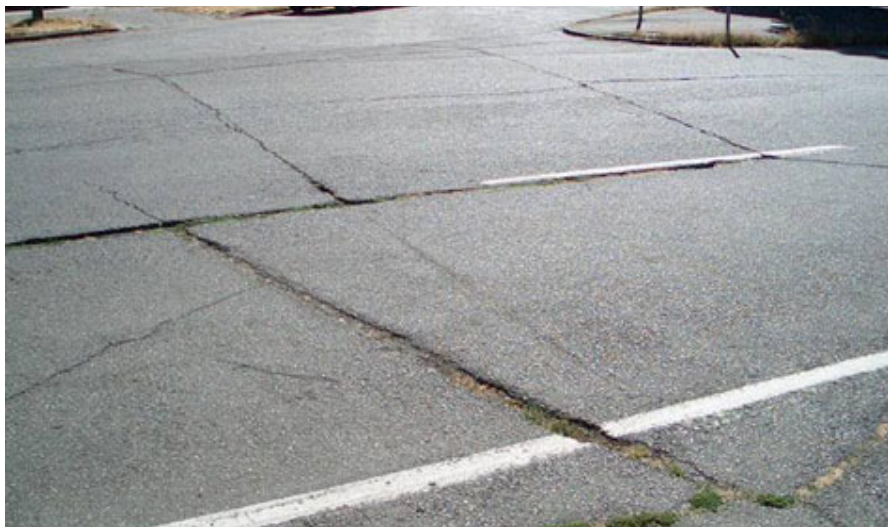
Figure 3.13 – Block cracking photo
