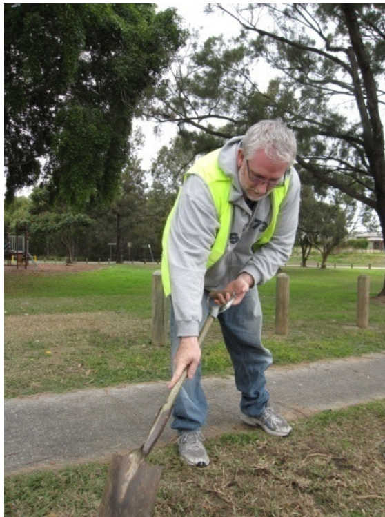
Figure 4.2 – Topsoil and turf removal with shovel
