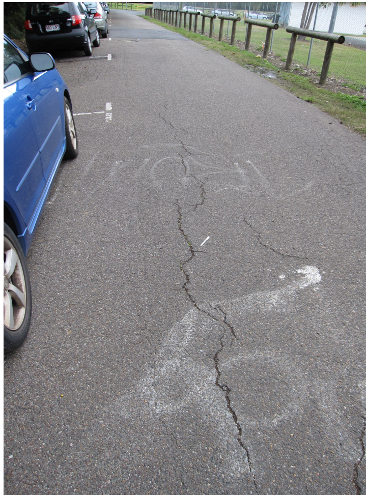
Figure 1.1 – Longitudinal cracking due to expansive subgrade
