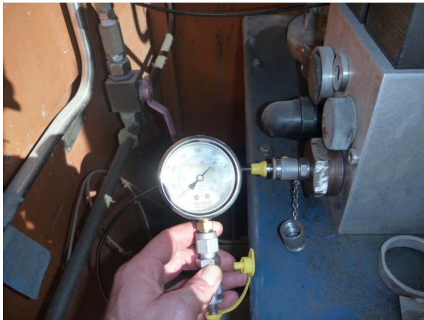
Figure 3.7: Individual pump pressure test
