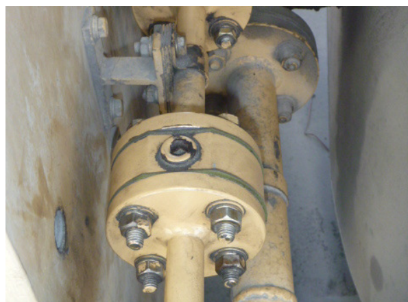
Figure 3.12: Adjustable orifice
