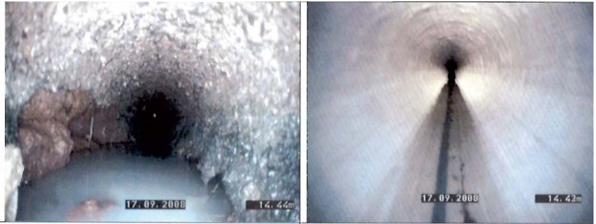
Figure 2-15 Example of sewer main pre and post cured in place relining (Insituform Pacific 2008)
