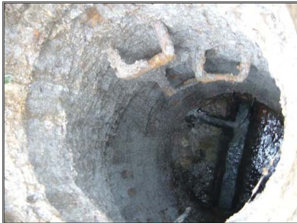
Figure 2-12 Example of concrete corrosion in a sewer maintenance hole
