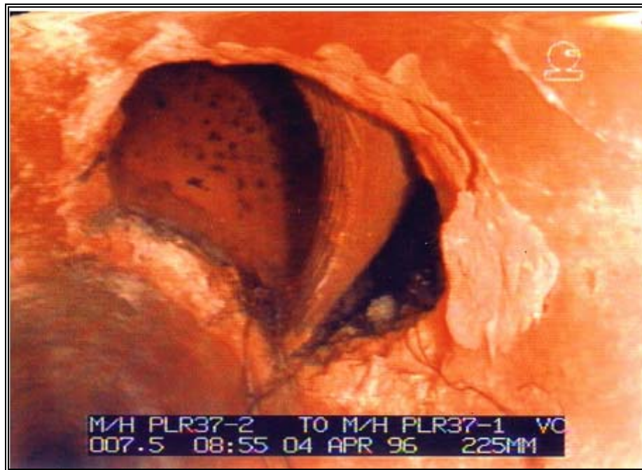
Figure 2-9 Example of poorly constructed lateral connection (WSAA 2005)
