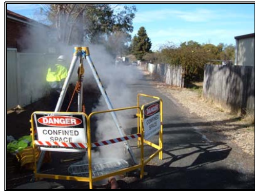
Figure 4-5 Sewer relining Ribloc (TRC 2010) Figure 4-6 Sewer relining cured in place (TRC 2010)
