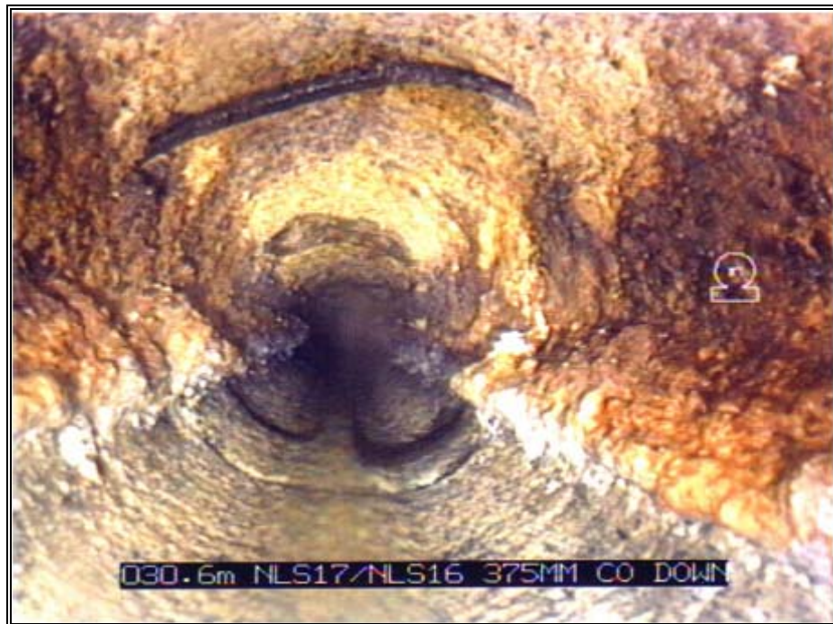
Figure 2-11 Example of concrete corrosion in a sewer main (WSAA 2005)
