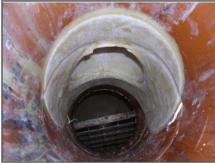
Figure 2-17 Example of sewer lateral connection lining (WSAA 2005)
