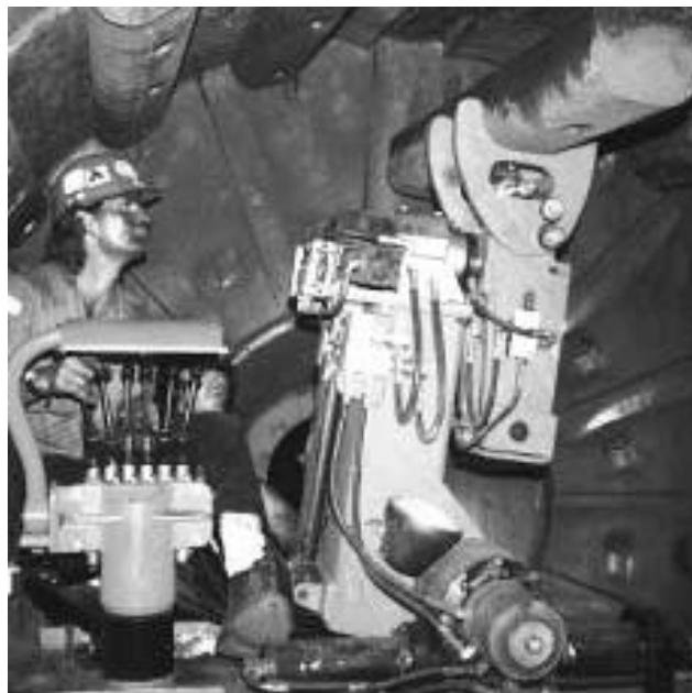
Figure 6.1: RME liner handling machine and operator (Source: http://www.rmeaus.com/ )
