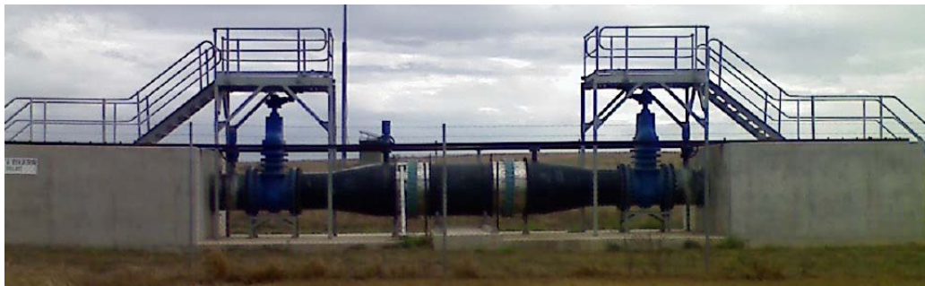
Figure 2.2 – Swab Structure on the Burdekin Moranbah Pipeline (SunWater 2005)
