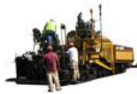
Figure 2.6: MILLIMETER GPS FOR PAVING
