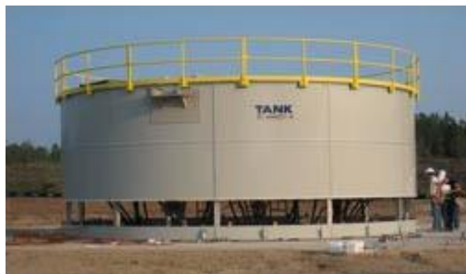
Figure 2.7 Hydraulic jack used in construction (Tank Connections 2009)
