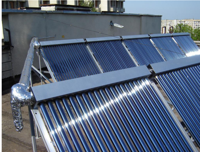
Figure 2.4 A sample ETC installation, (Source: Solar and wind energy, 2010)
