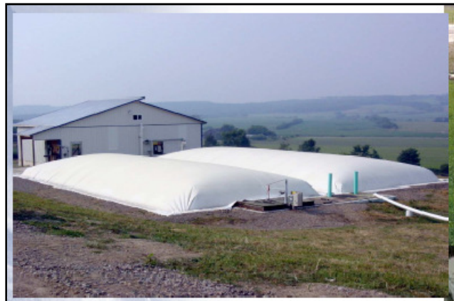
Figure 2-3 Example of an inflated pond cover
