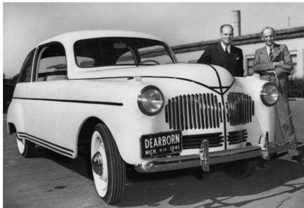
**Figure 3: The 1941 Ford which was made from Phenolic resin and hemp fibre**
