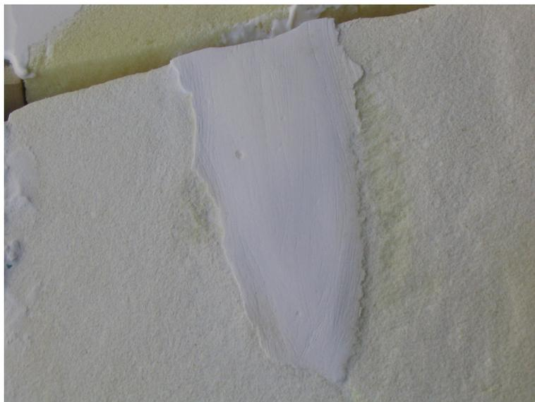
Figure 7.13: Close-up of a patch of bog, showing the eroded foam on each side.
