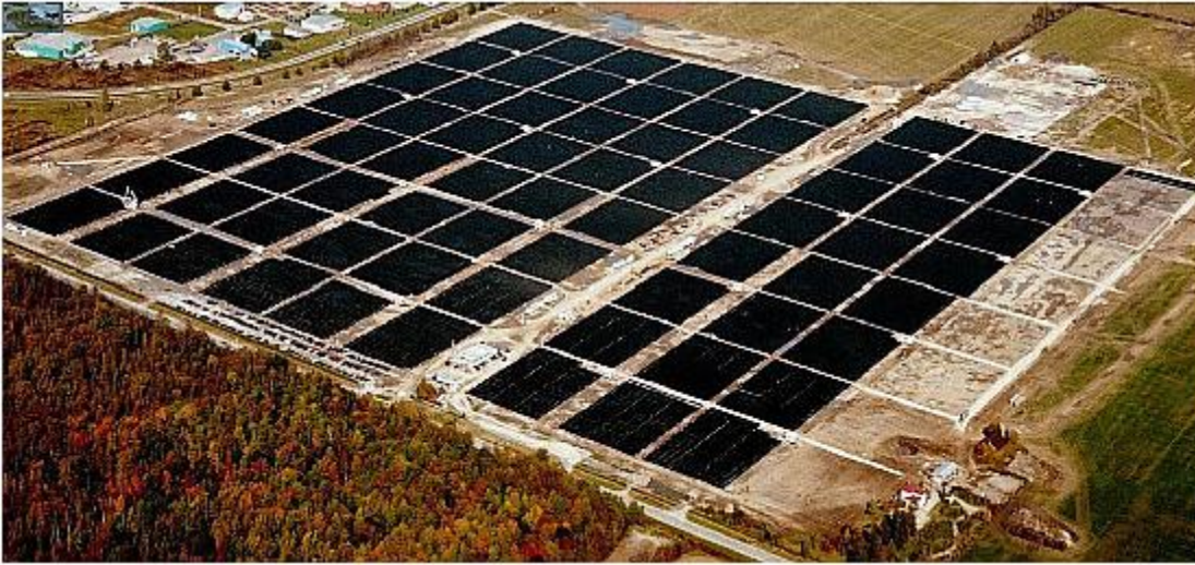
Fig 5.2 Sarnia Photovoltaic Power Station
