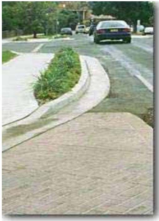
Figure 1.2: Application of Recycled Aggregate as Road Kerb (Source: Building Innovation & Construction Technology, 1999)
