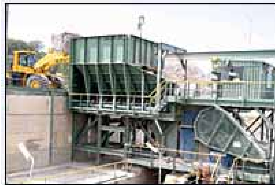
Figure 2.7: Load into Primary Crusher
