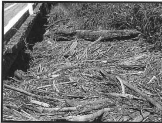
Figure 9 Flood Debris to be Removed
