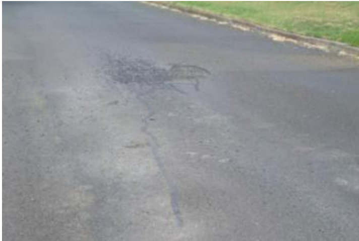
Figure 24 Teesdale Street – potholing (Sourced: TRC NDRRA Photo file 2011)
