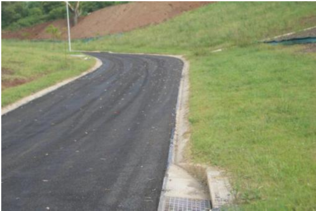
Figure 27 Anna Marie Street - restoration works - 'mill and fill'
