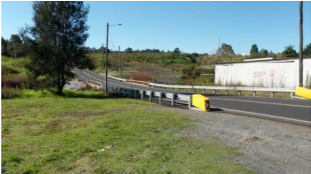
Figure 8 Griffith Street Bridge after Reconstruction
