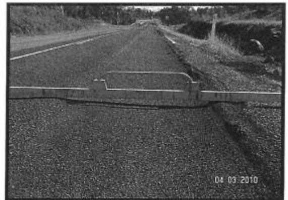
Figure 4 Pavement Rutting
