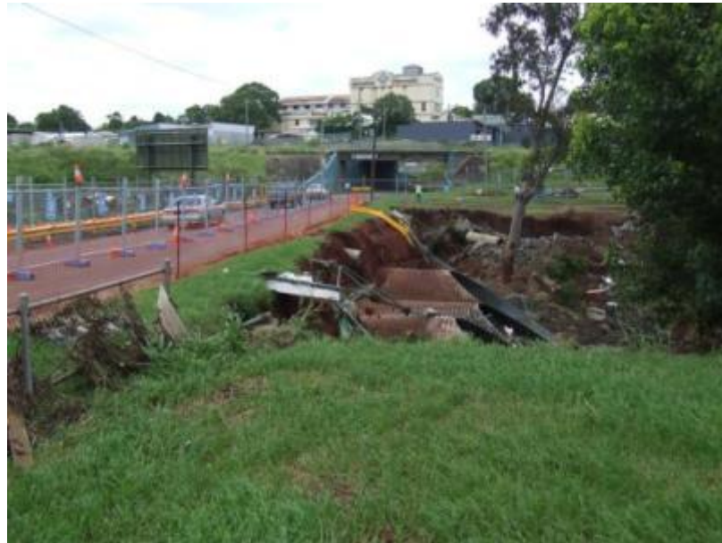
Figure 11 Bridge Street Culverts
