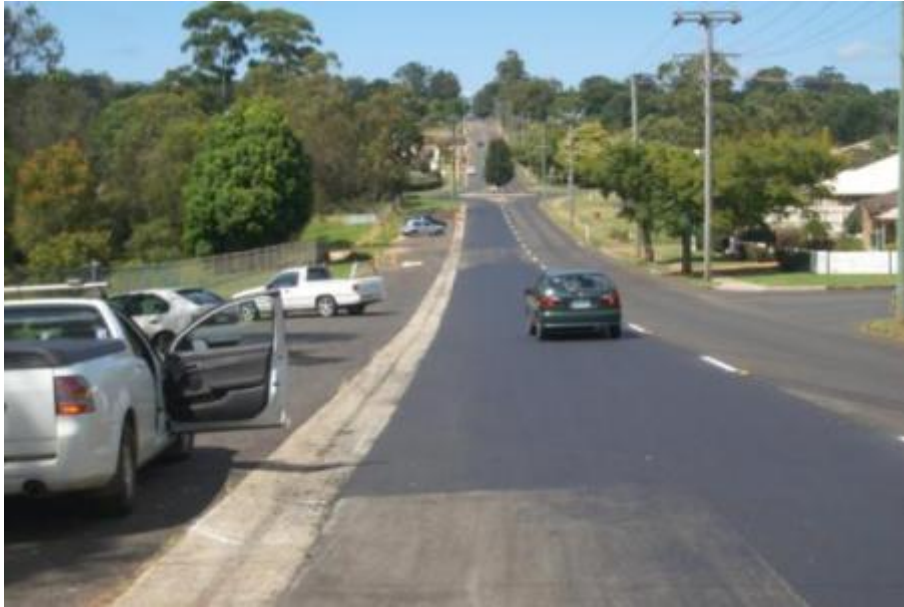
Figure 20 Mackenzie Street - restoration works - 'mill and fill'
