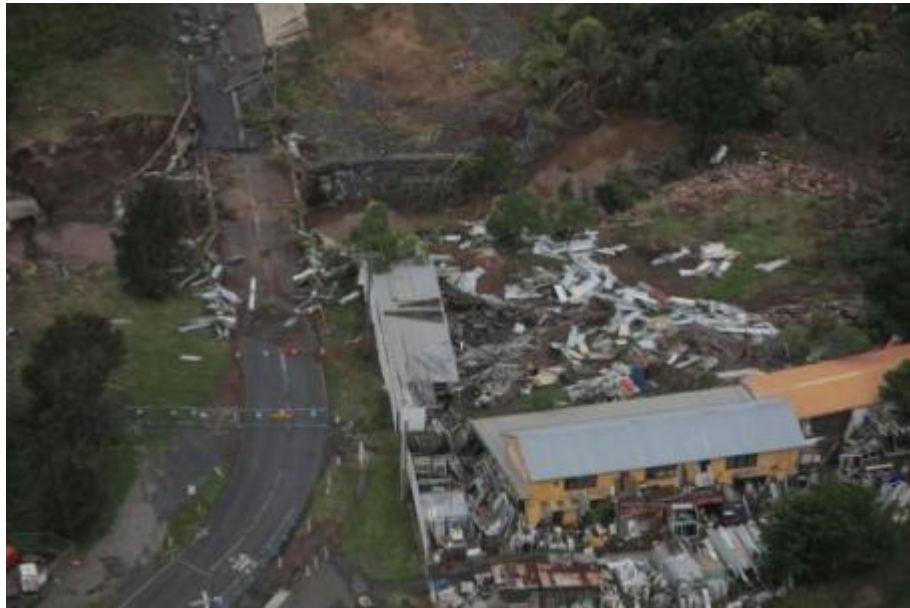
Figure 7 Griffith Street Bridge – Debris
