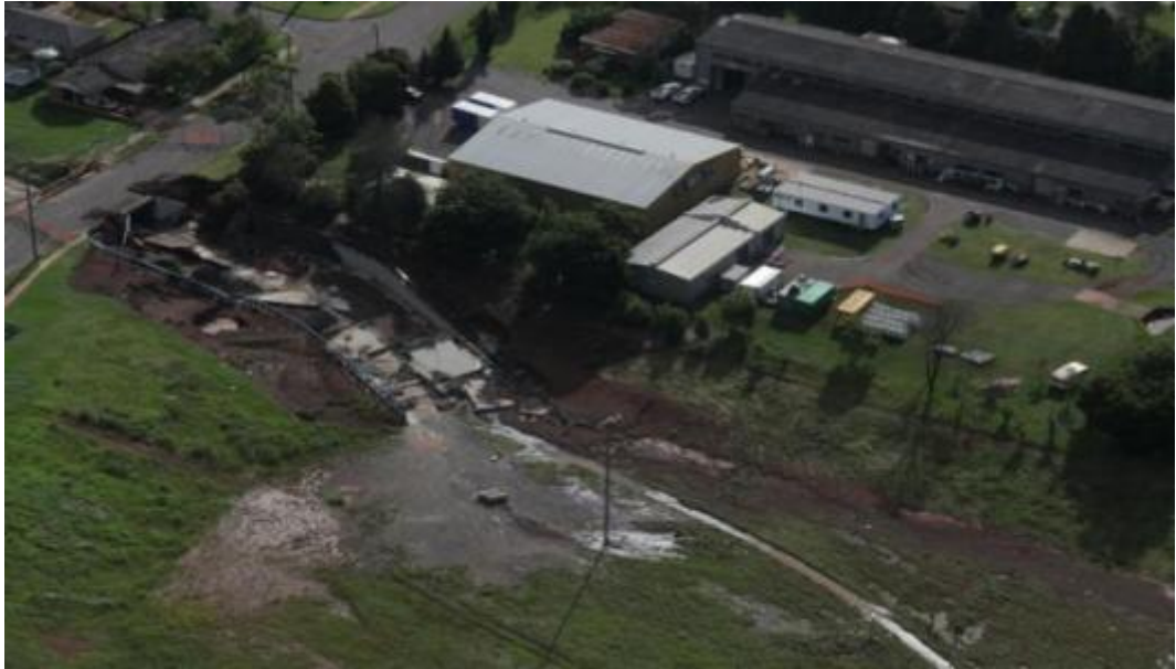
Figure 9 Wilf Gowlett Drop Structure South Street
