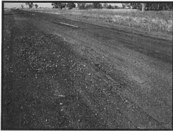
Figure 1 Pavement Breakouts
