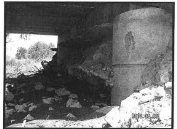
Figure 10 Scouring of Bridge Structures
