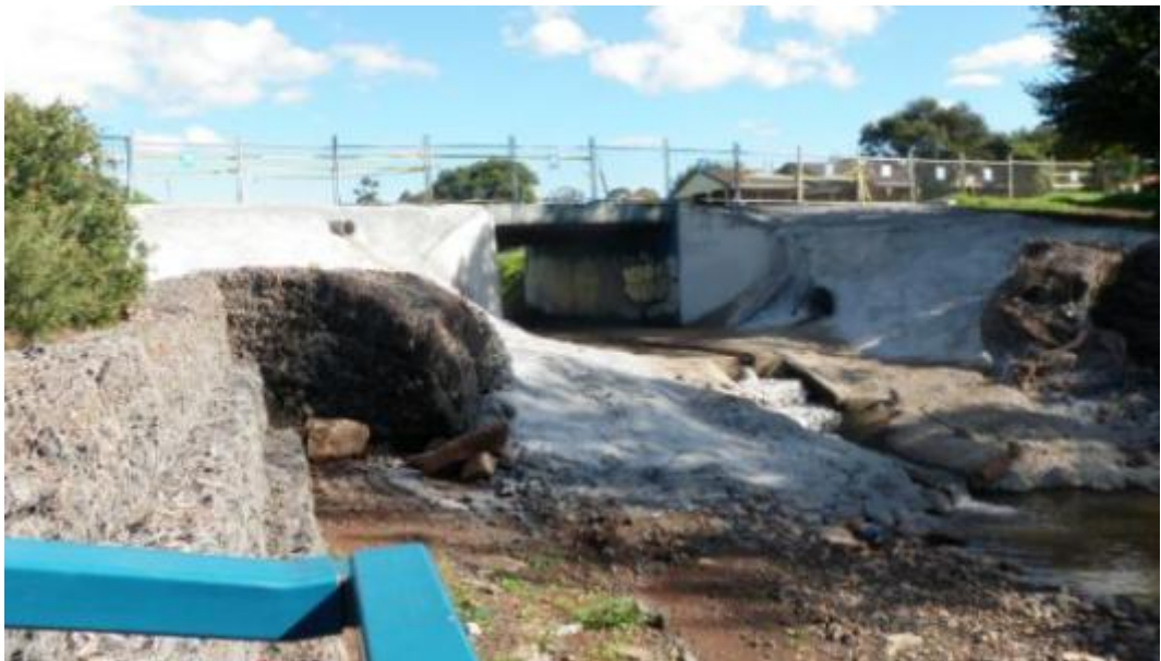
Figure 10 Wilf Gowlett Drop Structure after Reconstruction
