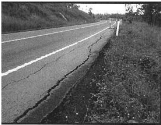
Figure 15 Embankment Slump
