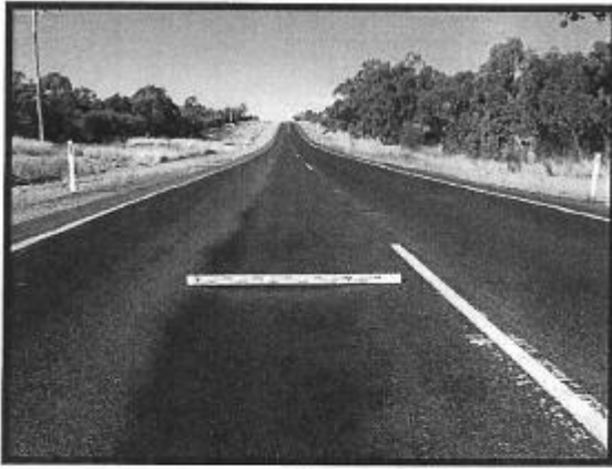
Figure 7 Flushing of Bitumen Seal in Wheel Paths
