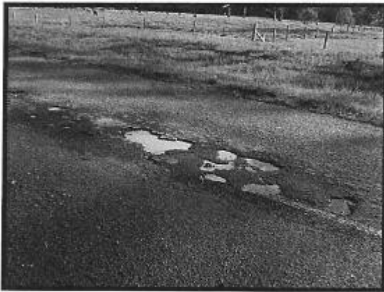
Figure 3 Pavement Potholing
