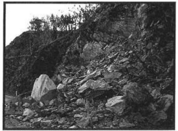
Figure 14 Slope Failure & Instability
