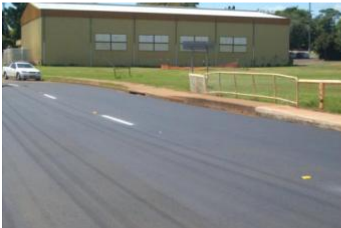
Figure 22 South Street - restoration - 'mill and fill'
