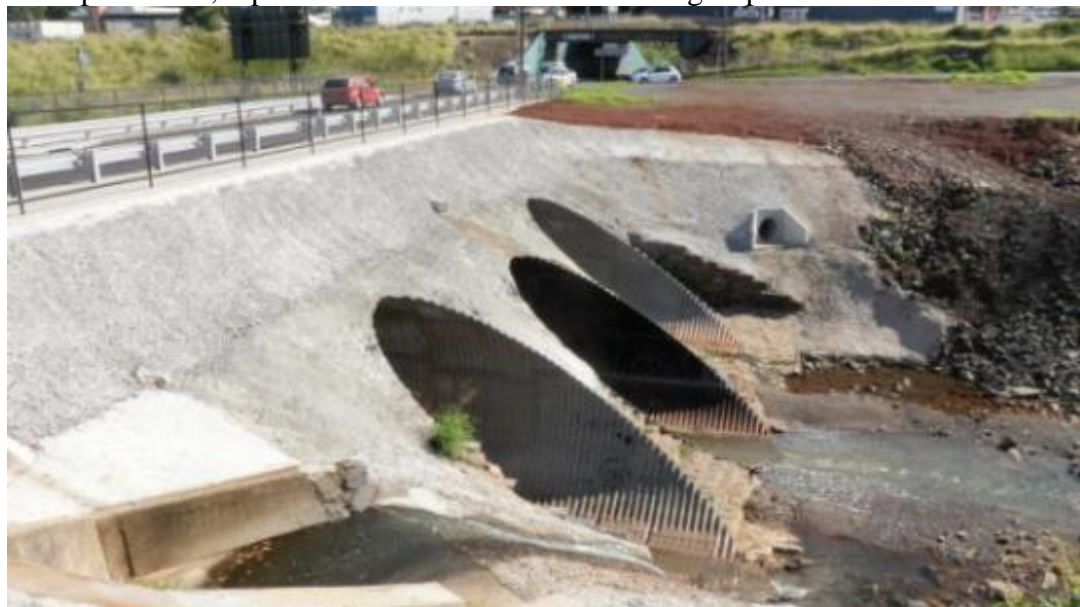
Figure 12 Bridge Street Culverts after Reconstruction
