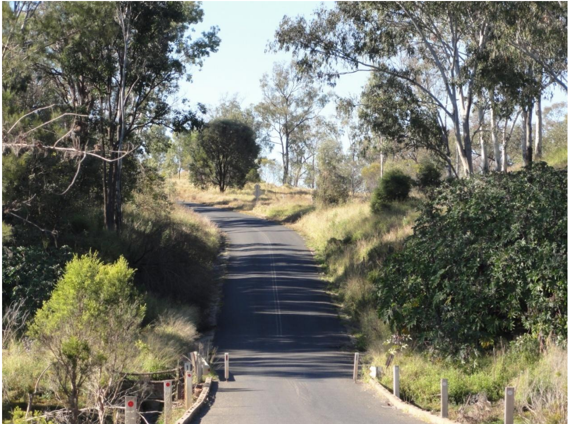
Figure 25: The approach to Jack Parr Bridge from Mundubbera
