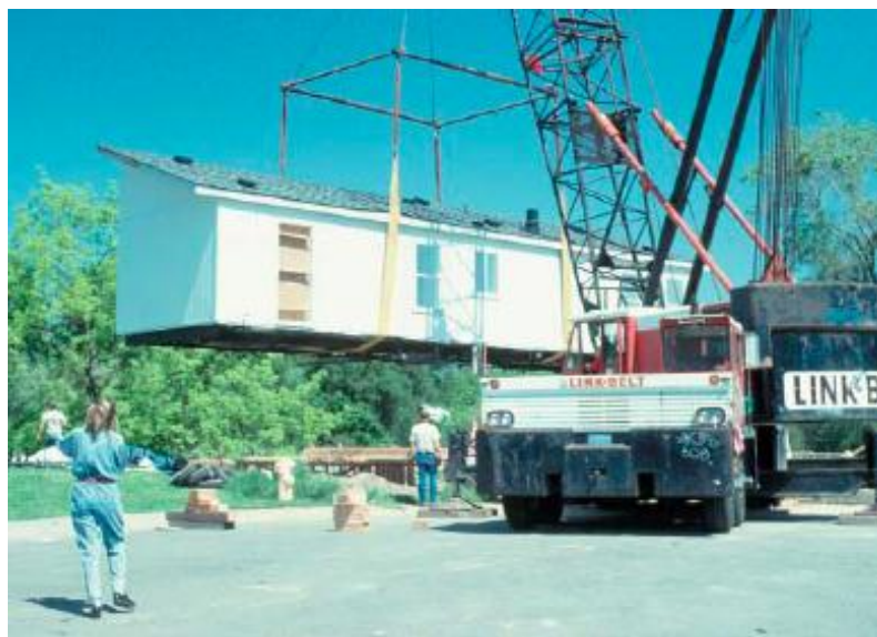
Figure 2.5 – House Craned into Position (MHRA, 2002)
