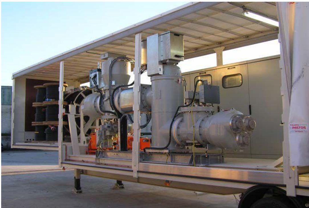
Figure 20: A typical GIS switchgear (Ergon Energy, 2011)
