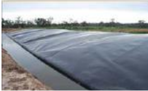
Figure 3.2: Covered anaerobic pond at Churchill Abattoir
