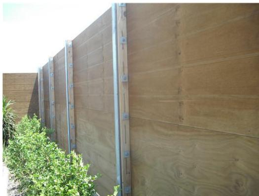
Figure 5 Plywood noise barrier (<http://www.fhwa.dot.gov/environment/keepdown.htm>)
