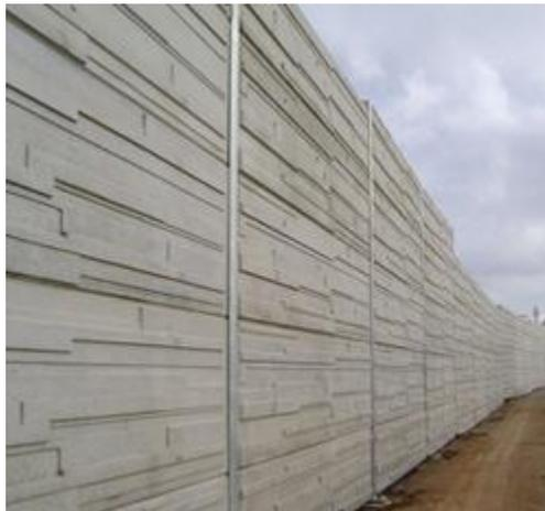
Figure 2 Concrete Noise barrier ([http://noisebarriers.com.au/noise\\_barriers\\_portfolio.php](http://noisebarriers.com.au/noise_barriers_portfolio.php))
