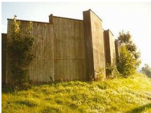
Figure 6 Glue laminated noise barrier (<http://www.fhwa.dot.gov/environment/keepdown.htm>)
