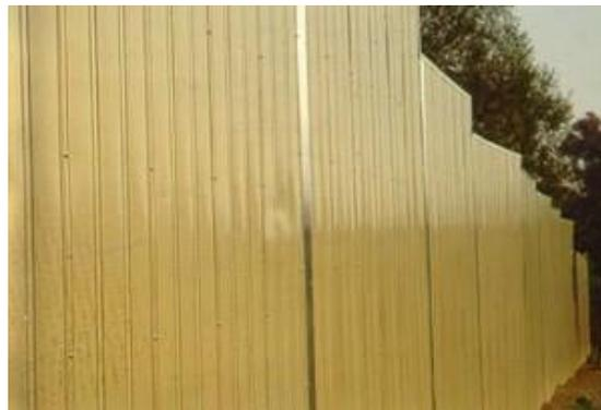
Figure 4 Aluminium noise barrier ([http://noisebarriers.com.au/noise\\_barriers\\_portfolio.php](http://noisebarriers.com.au/noise_barriers_portfolio.php))
