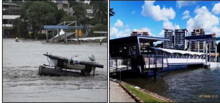
Figure 4-18 Sydney St before and after
