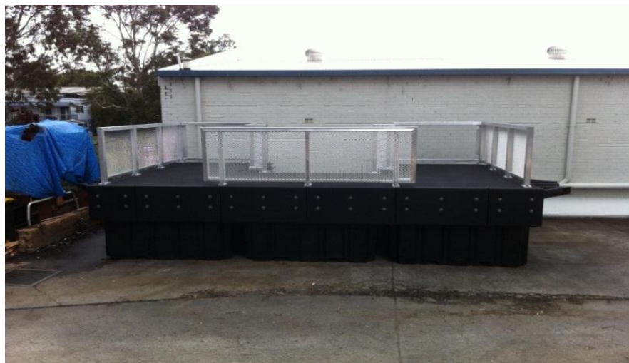
Figure 4-16 Constructed QUT pontoon
