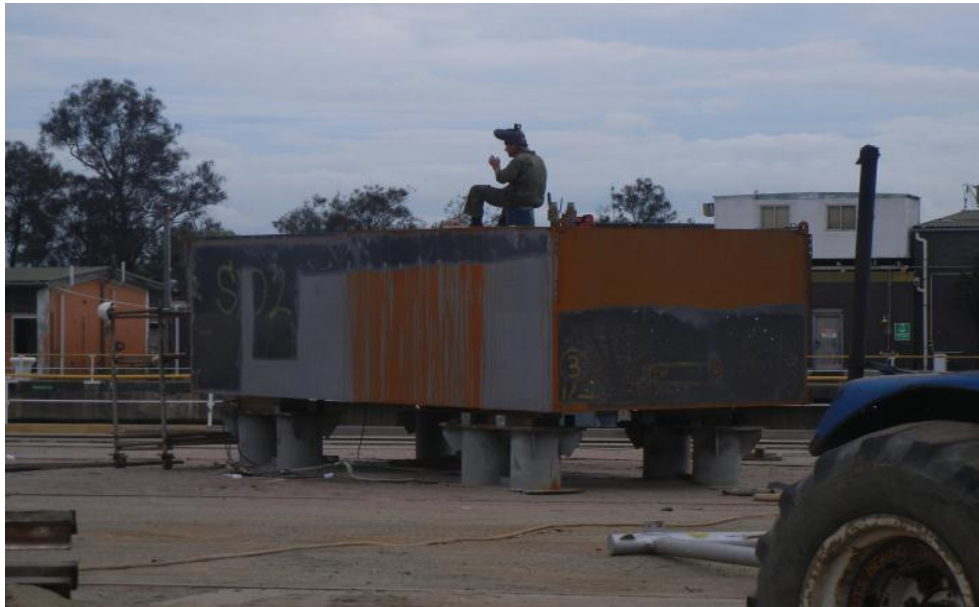
Figure 4-12 Pontoon section being repaired
