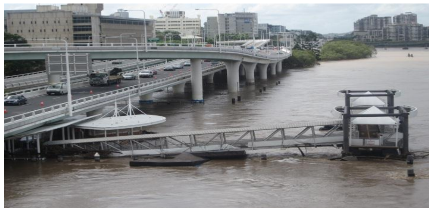
Figure 1-2 North Quay Passenger terminal during 2011 flood
