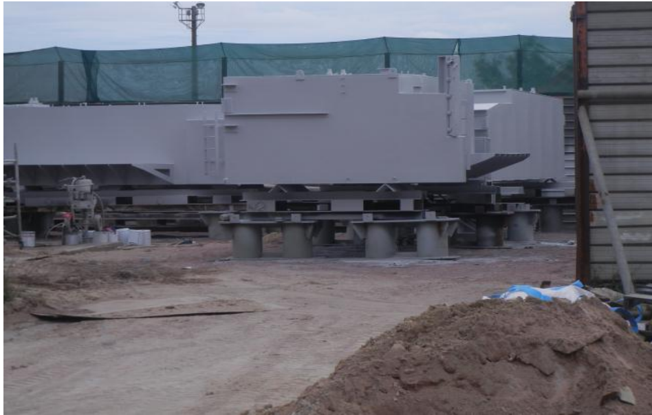
Figure 4-13 Pontoon sections being painted
