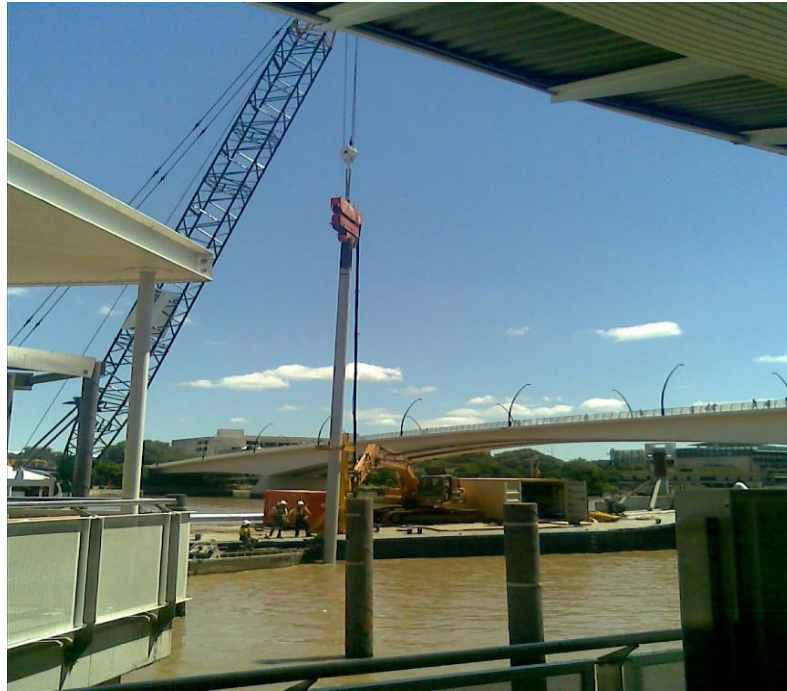
Figure 4-14 Vibrating pile into place at North Quay
