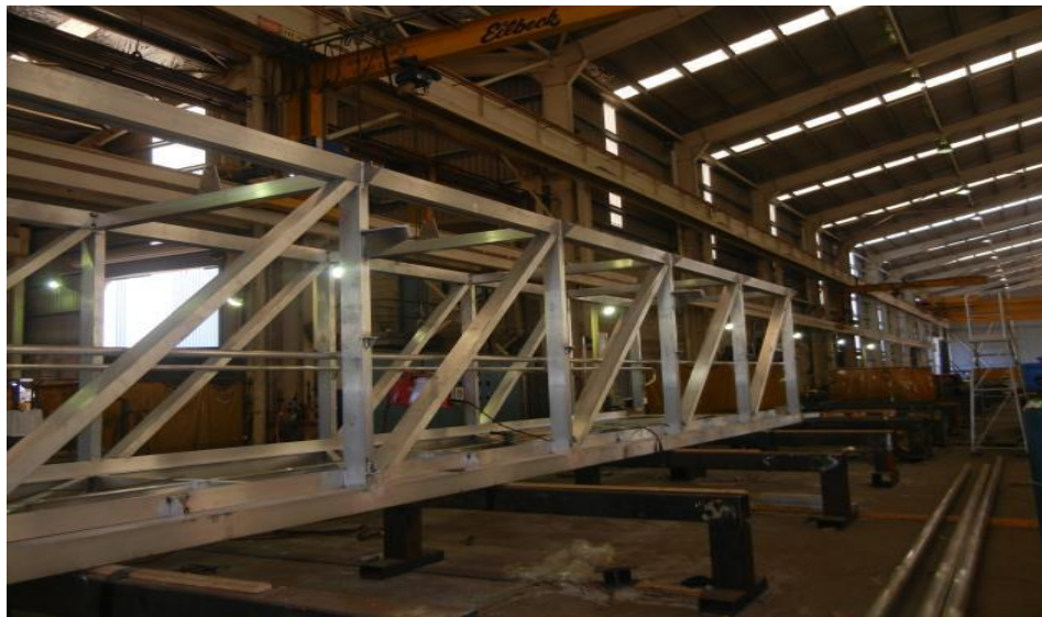
Figure 4-8 Gangway construction in Sydney workshop
