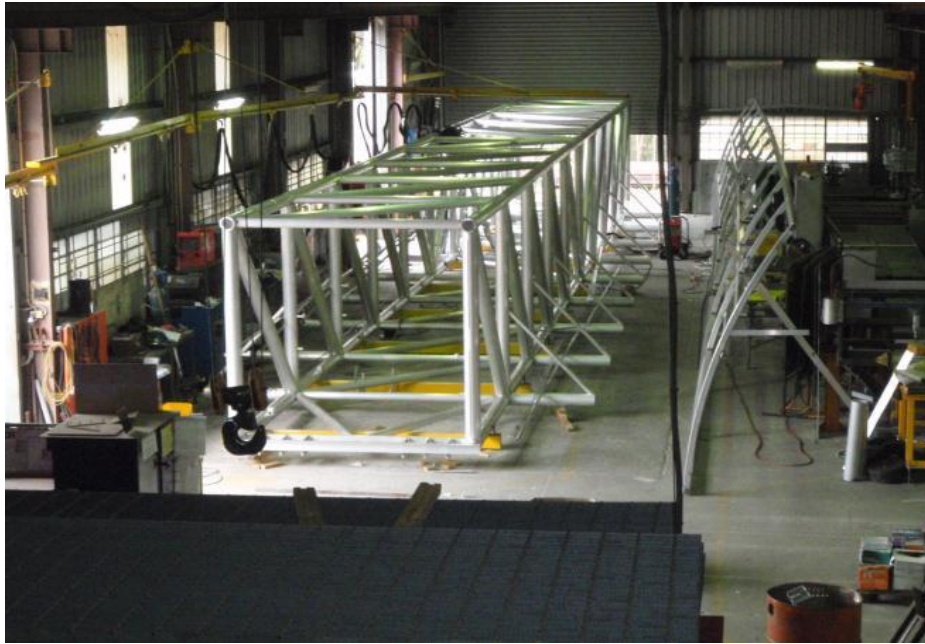
Figure 4-9 Gangway construction in Brisbane workshop
