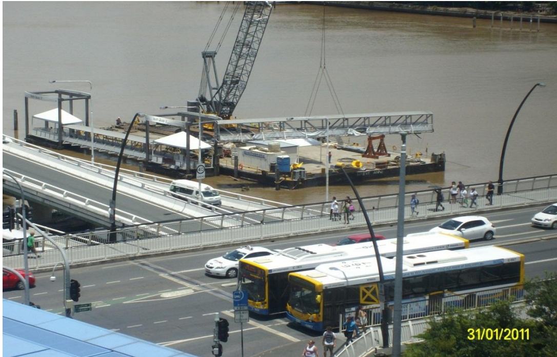
Figure 4-3 519 Tonne Crane Barge 'Maeve Anne' removing Gangway from North Quay
