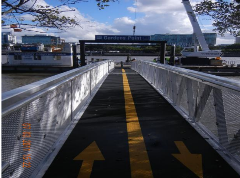
Figure 4-17 QUT Gangway in position
