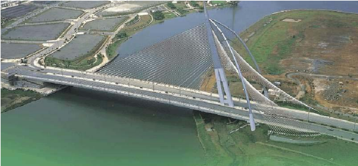
Source: Putrajaya Bridge Construction Team, 2005
