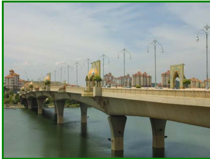
Source: Putrajaya Bridge Construction Team (2005)
