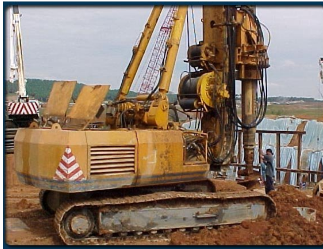
Source: Putrajaya Bridge Construction Team (2005)
