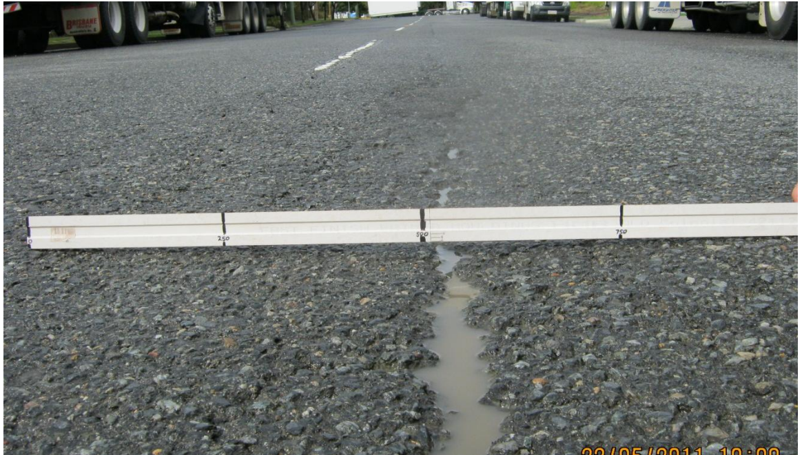
Figure 4-3: Longitudinal cracking at Darra
