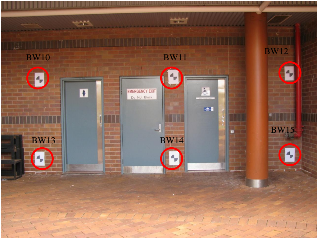
Figure 3.2-4: USQ TLS calibration range West wall BW targets only
