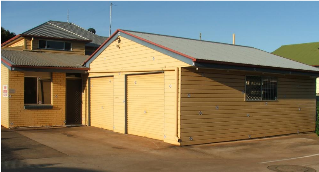
Figure 3.8 Outdoor Building Site (Site 2)
