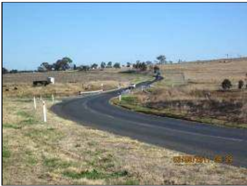
Figure 6.6: Crash site 1 Clifton-Leyburn Road looking north-west
