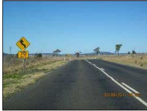
Figure 6.18: Crash Site 3 Toowoomba-Karara Road, crest leading into horizontal curves
