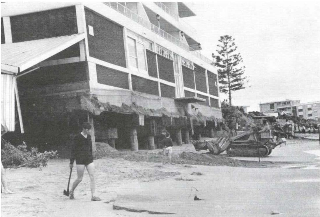
*Figure 19* – ‘Flight Decks’ exposed foundations after 1967 storm (Worley Parsons 2011)
