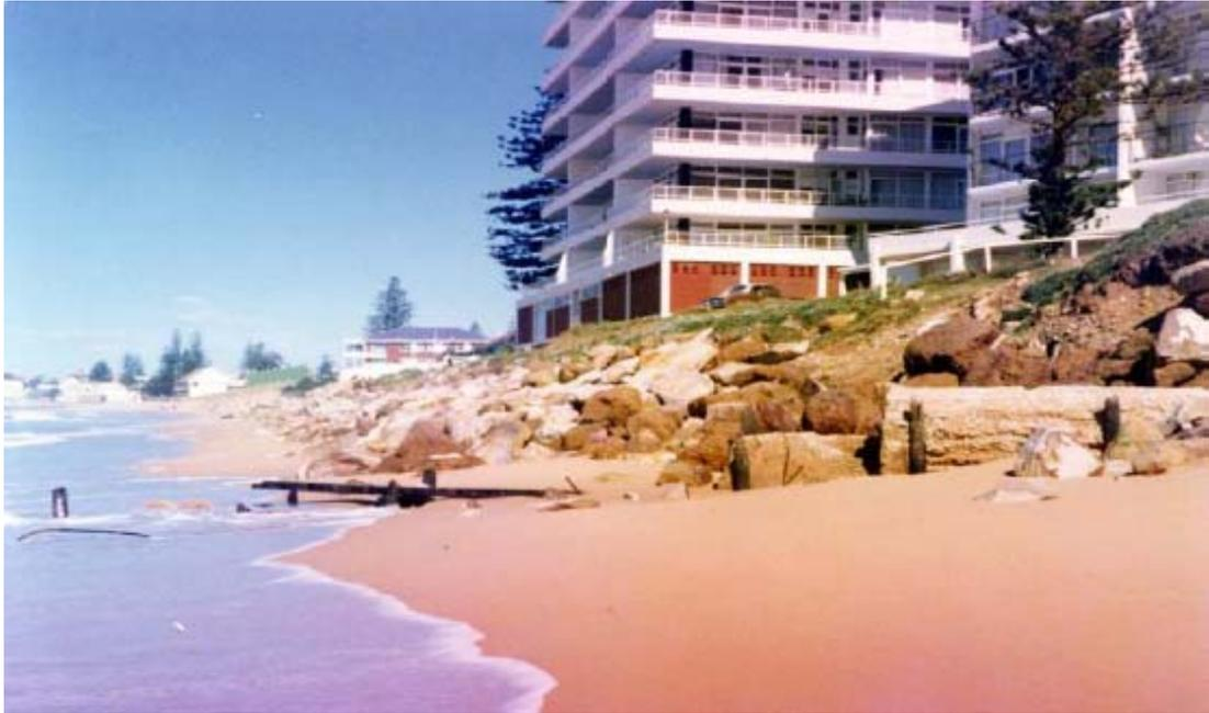
*Figure 27 – Emergency rock protection in front of ‘Shipmates’ & ‘Flight Deck’ c.1972 (Worley Parsons 2011)*
