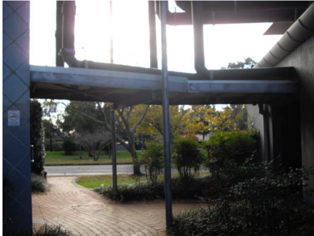
Figure. 3.9 The bridge structure showing where the simulation was conducted.
