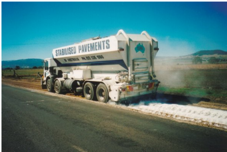
Figure 3.1 Lime Spreading on Widening to Cunningham Highway Trial Project
