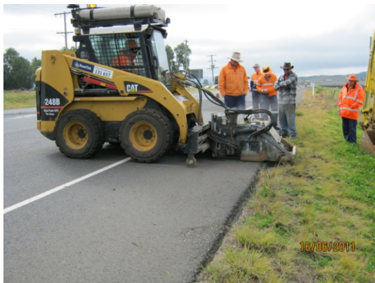
Figure 3.7: Asphalt Excavation
