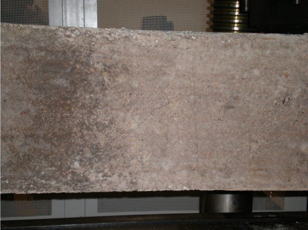
Photo 9 – Initial cracking in conventional beam
