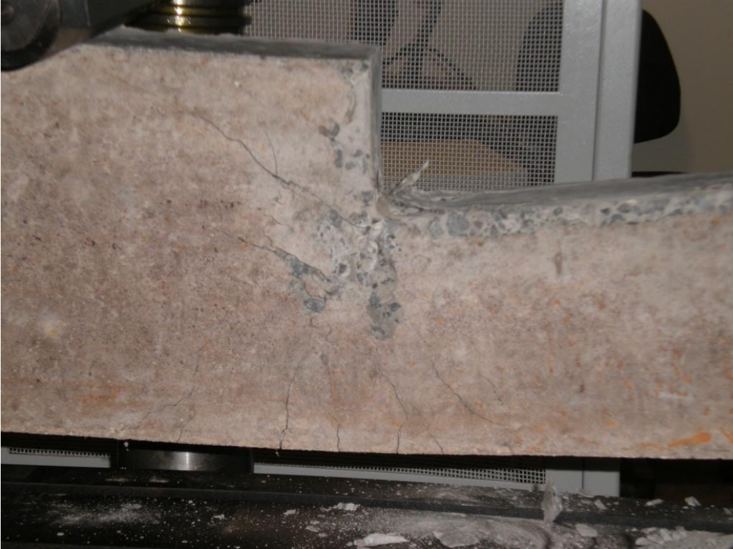
Photo 10 – Initial cracking in conventional beam at depth discontinuity
