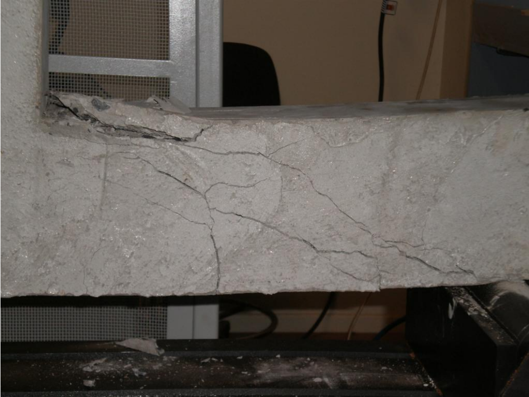
Photo 6 – Further cracking in the optimum beam
