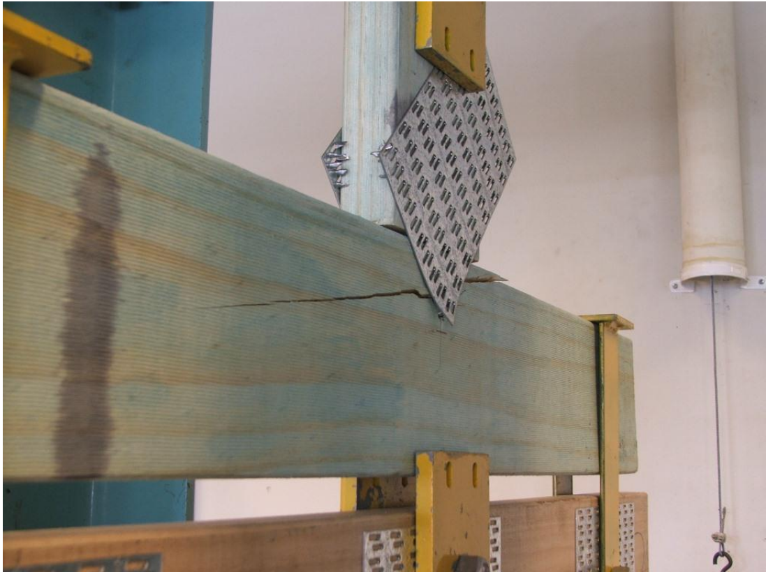
Figure 4.18 - Tension perpendicular failure even after plate withdrawal
