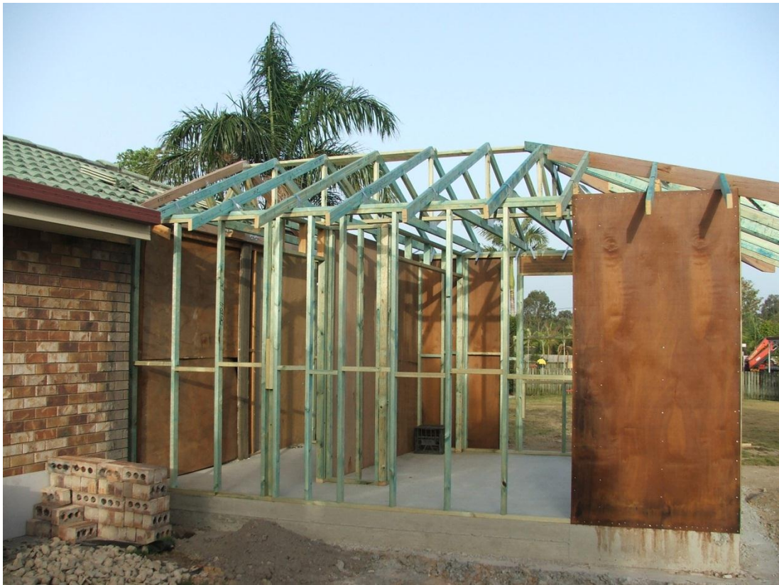
Figure 1.1 - Roof Trusses in use (during construction)
