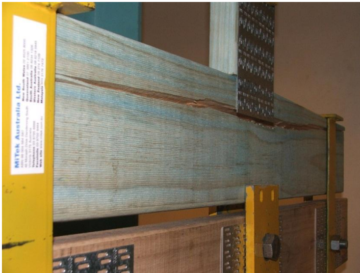
Figure 4.1 - ID5 Failure at bottom row of teeth
