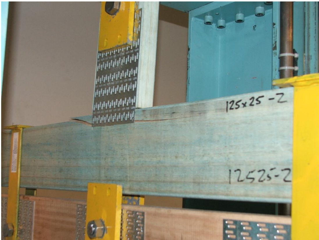
Figure 4.4 - Small fracture length along grain
