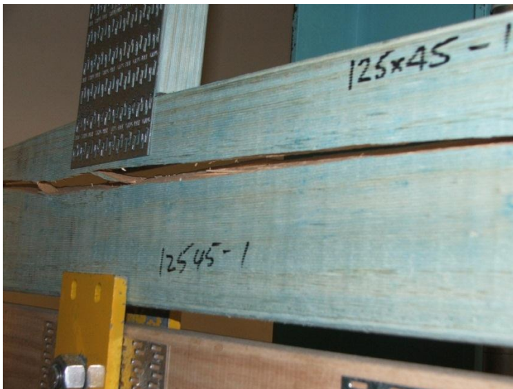
Figure 4.2 - ID5 failure below the plate
