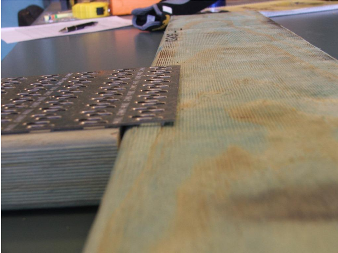
Figure 4.6 - Timber fibres failure laterally with appearing like plate withdrawal
