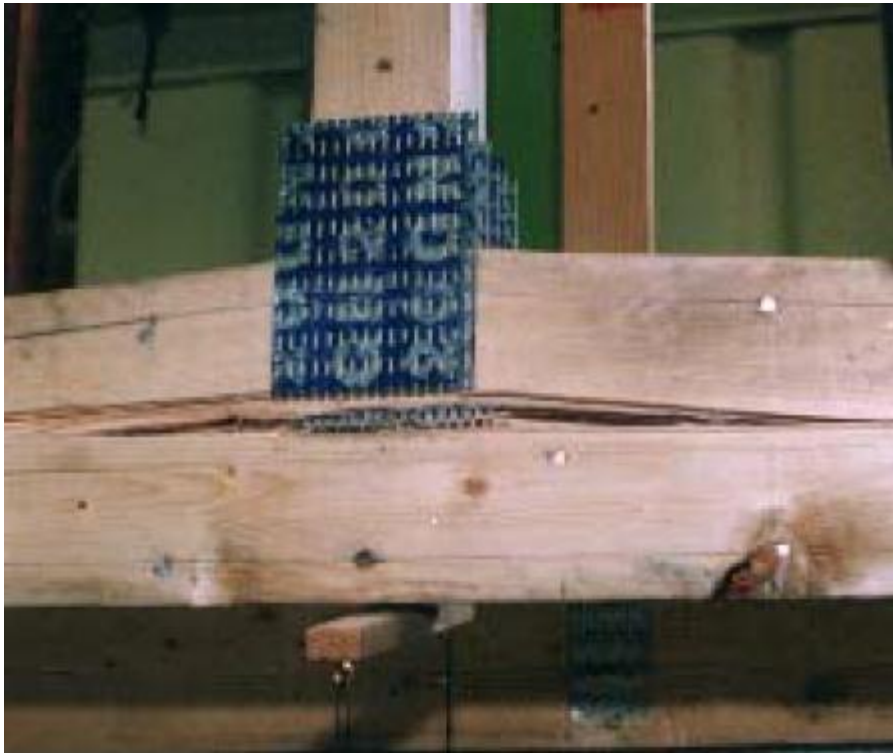
Figure 2.2 - Common Tension Perpendicular Failure (Enjily, 2001)
