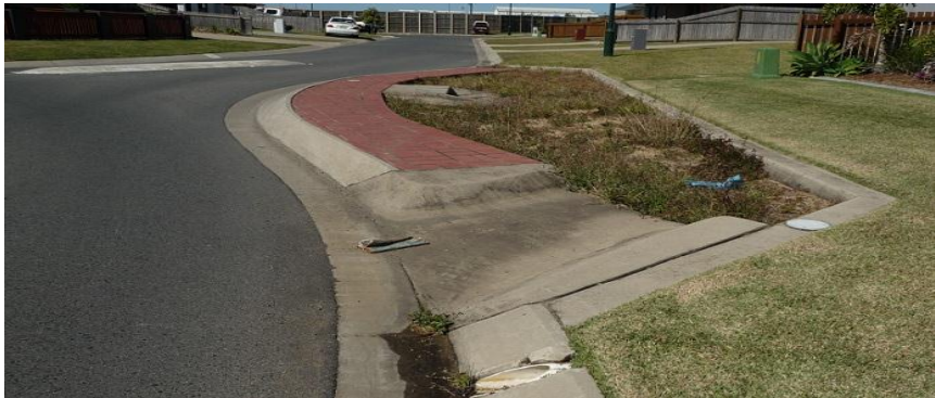
Fig. 4-17: An example of an unmaintained biopod located in Cuttersfield that contains weeds and rubbish.
