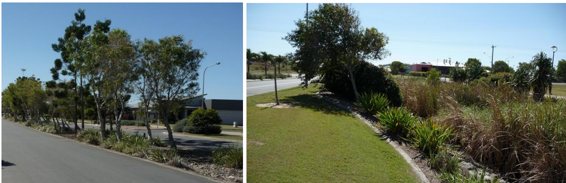
Fig. 2-3: Typical central boulevard bioretention swale, Cuttersfield Mackay (left) and bioretention basin Blacks Beach (right), Mackay.
