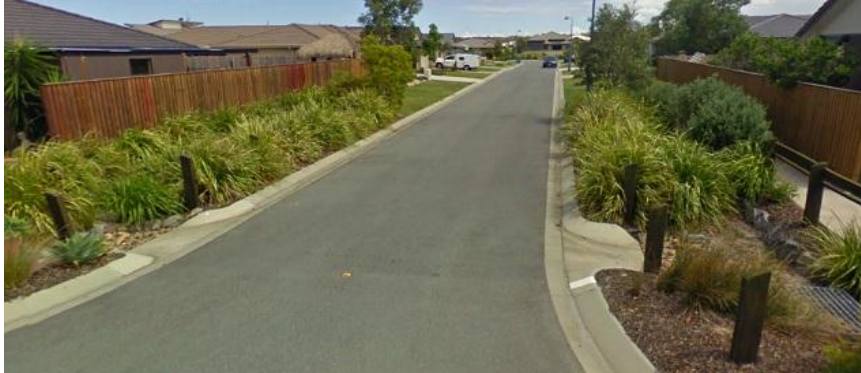
Fig. 4-18: An example of a fully planted and maintained biopod, Bellvista Estate, Caloundra, Google Maps (2012).
