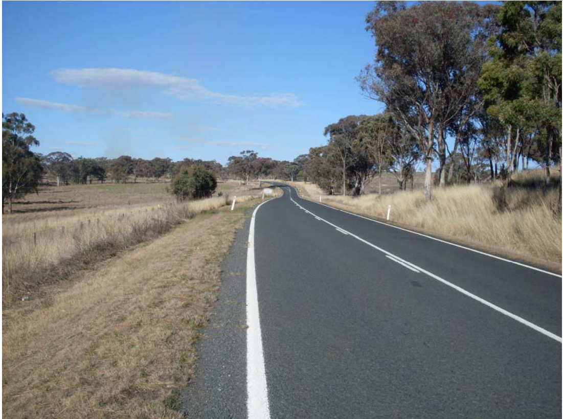
Figure 4.7 Gwydir Highway at Elsmore site
