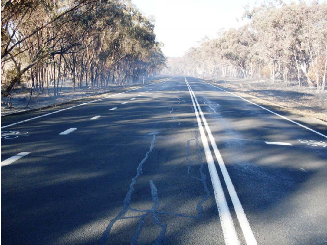
Figure 5.26 Gwydir Highway at Elsmore showing crack sealing
