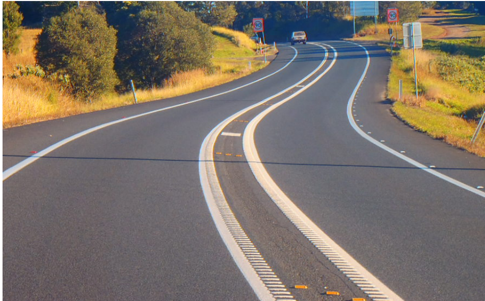
Figure 1.5: Continuous Painted Median Strip Installation
