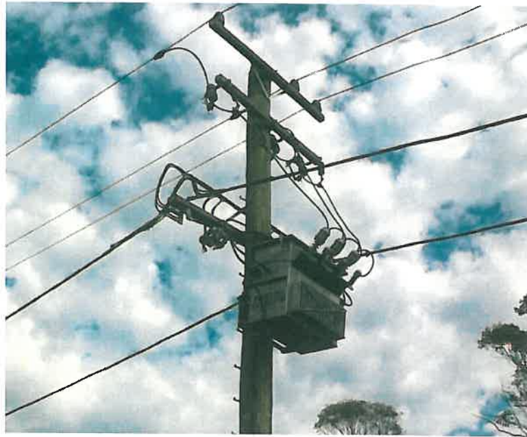
Figure 3: Photo of an in-service ASC Pole Top Transformer Currently on Trial
