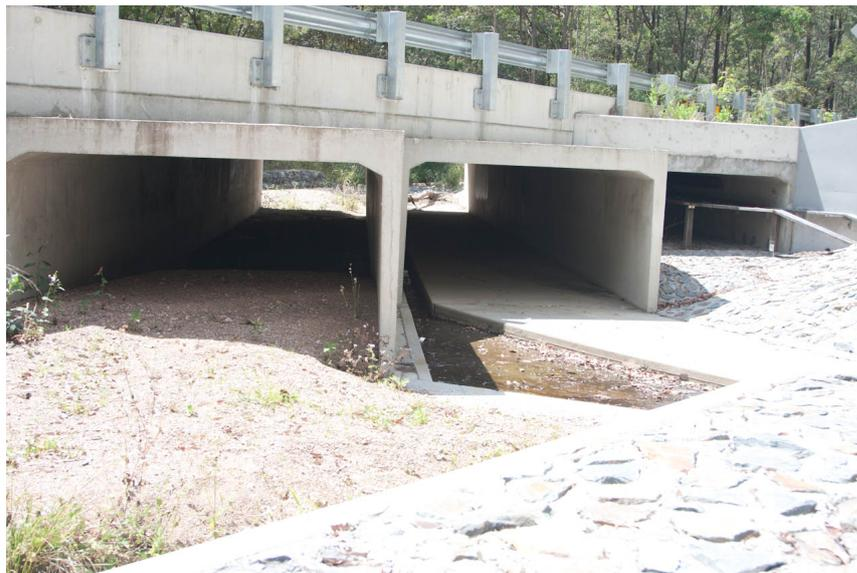
Figure 1.1: Wildlife crossing tunnels developed at Gap Creek Road, Pullenvale. Source: Ashton Fagg
