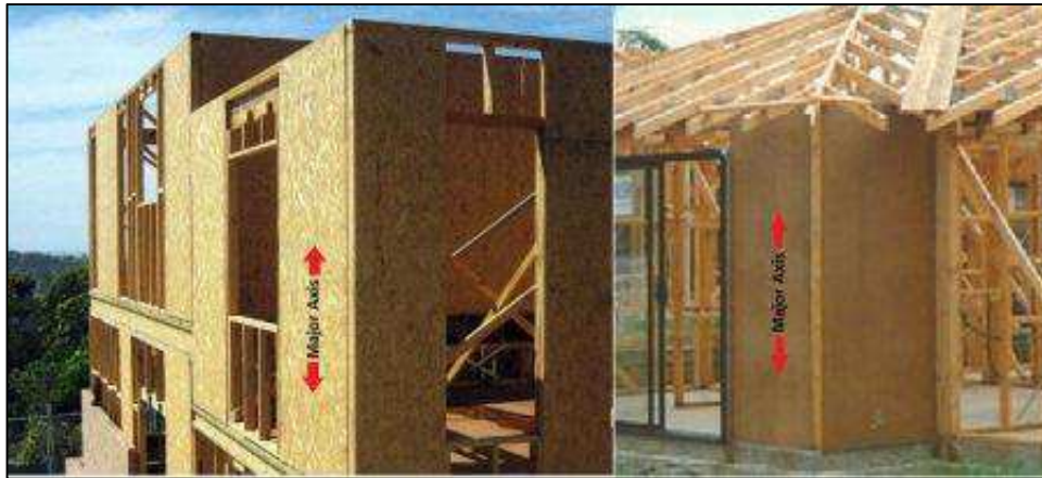
Figure 3.3: OSB and Plywood bracing panels with major axis in vertical direction
