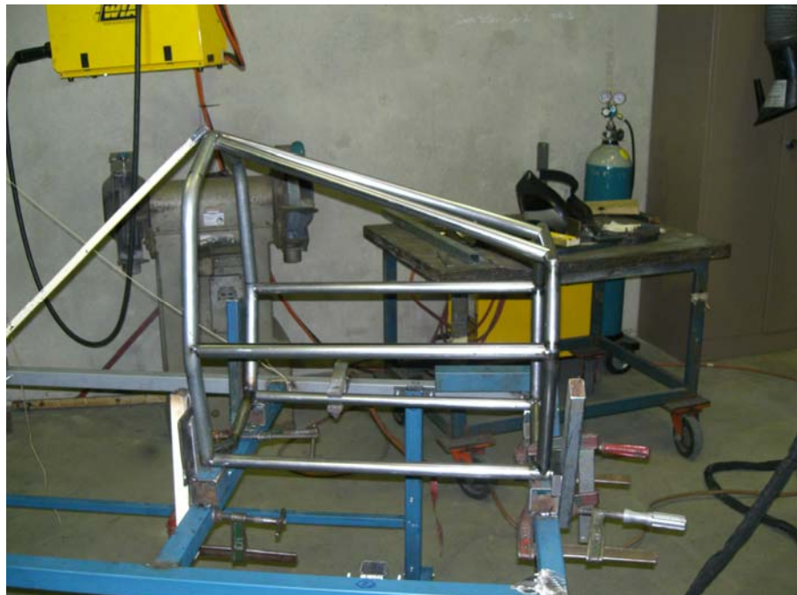
Figure 44: First pipes to be added to the main components the front supports.
