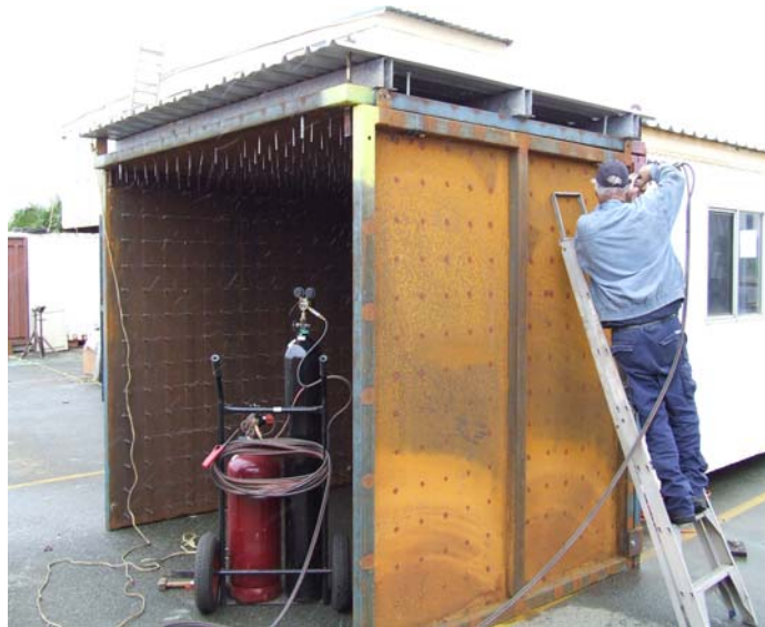
Overall view of partial assembly
