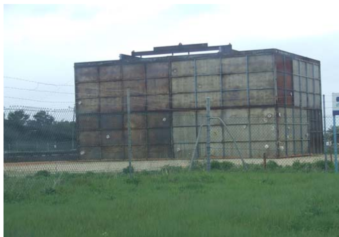
Figure 1.1- Large gas fired stress relieving furnace
