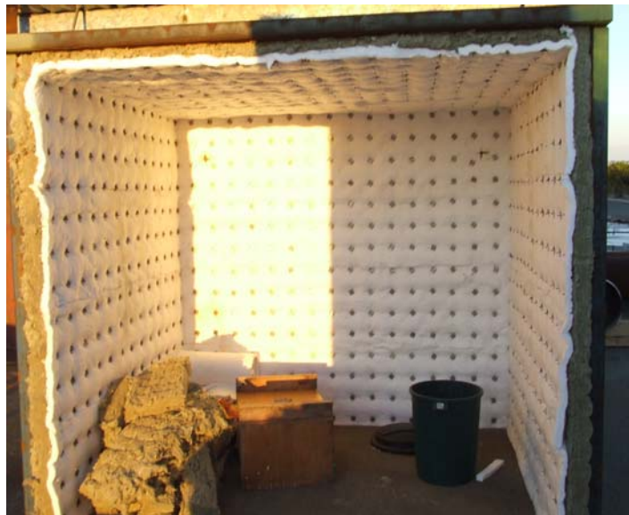
Partial Assembly showing refractory pins
