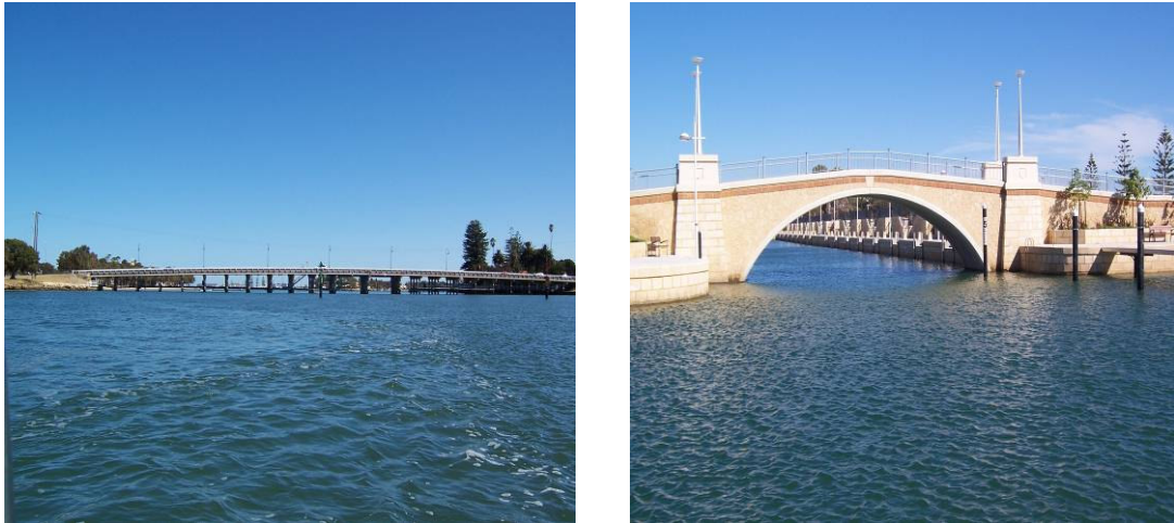
Figure 4-3 Typical Bridge Infrastructure Assets
