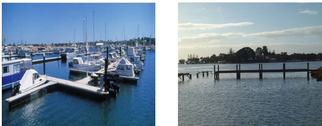
Figure 4-6 Typical Coastal and Marine Infrastructure Assets
