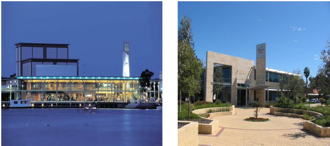
Figure 4-5 Typical Building and Facilities Infrastructure Assets
