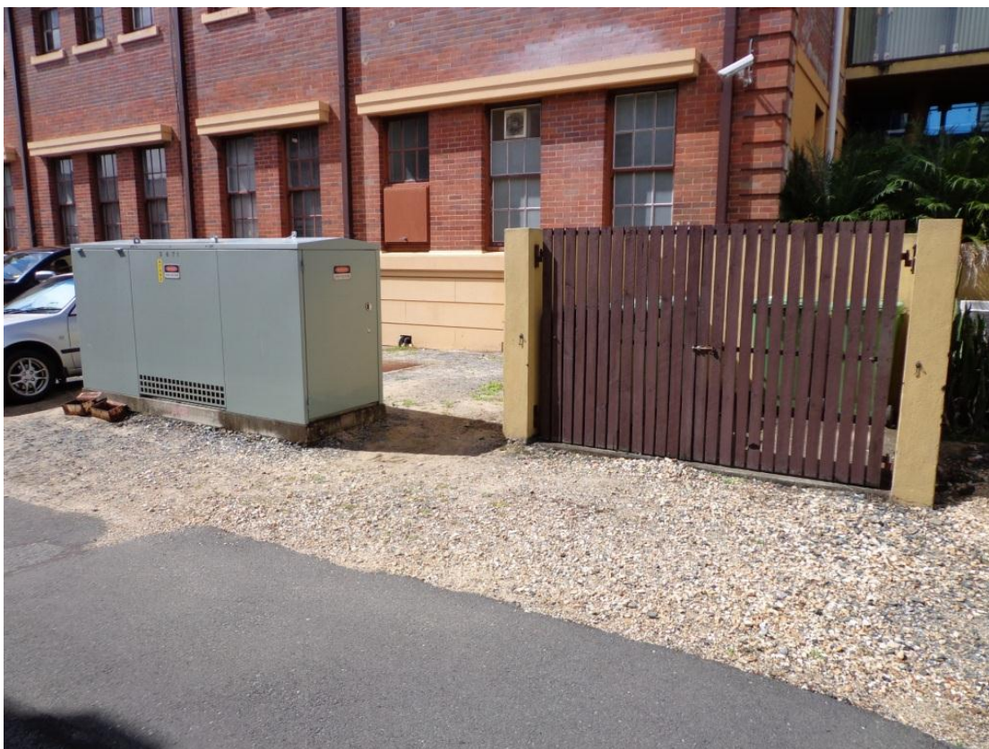
Pad mounted transformer and bin storage in Tenth Lane
