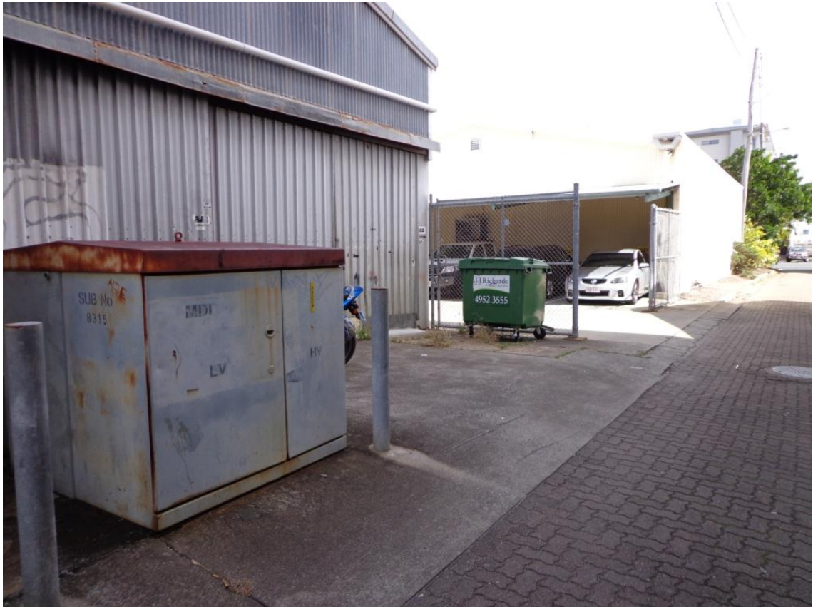
Figure 4.4 A pad mounted transformer in Second Lane
