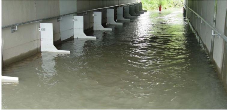
Figure 8.4: Corner 'EL' Baffle - Culvert Barrel (Kapitzke 2007)
