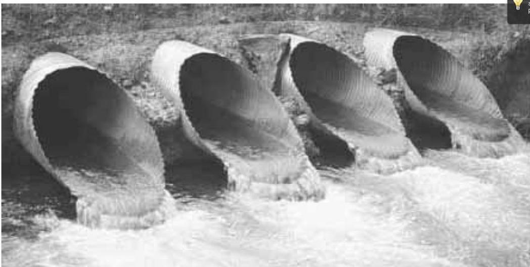
Figure 4.1: Perched culvert outlet as a result of erosion (Cotterell 1998)
