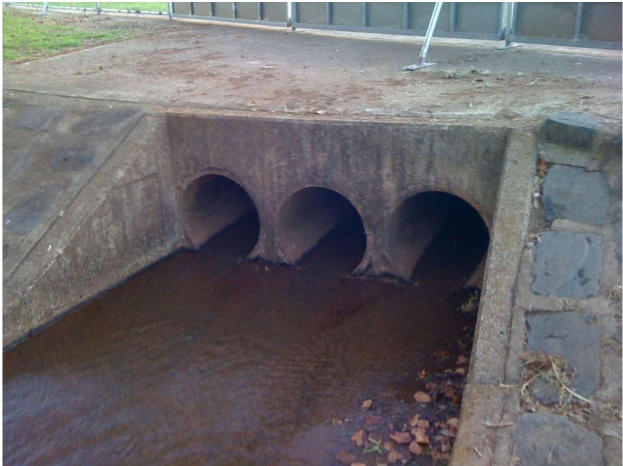
Figure 3.1 – Outlet of culvert under McKenzie St, discharging into WBH
