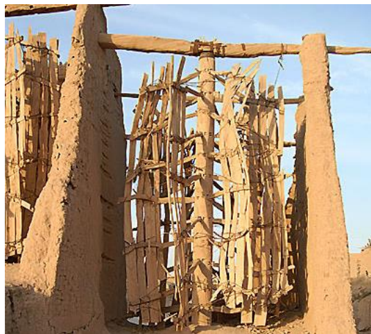
Figure 1.2a Early Persian vertical grain milling machine, 7 th century design (Shahmiri 2009)
