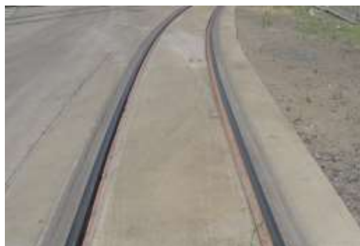
Figure 4-4: Pre- concrete cutting
