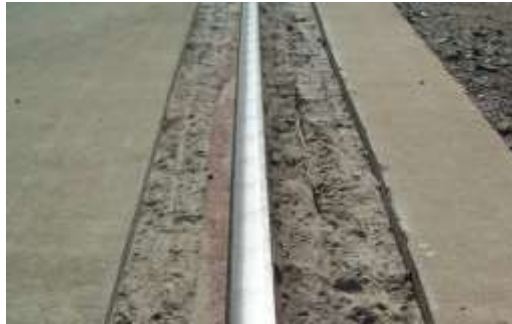
Figure 4-5: Post concrete cutting
