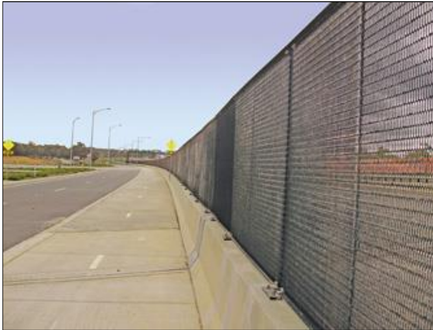
Figure 2.21: Ingal Civil Products Headlight Dazzle Screen Source: (Ingal Civil Products 2013)
