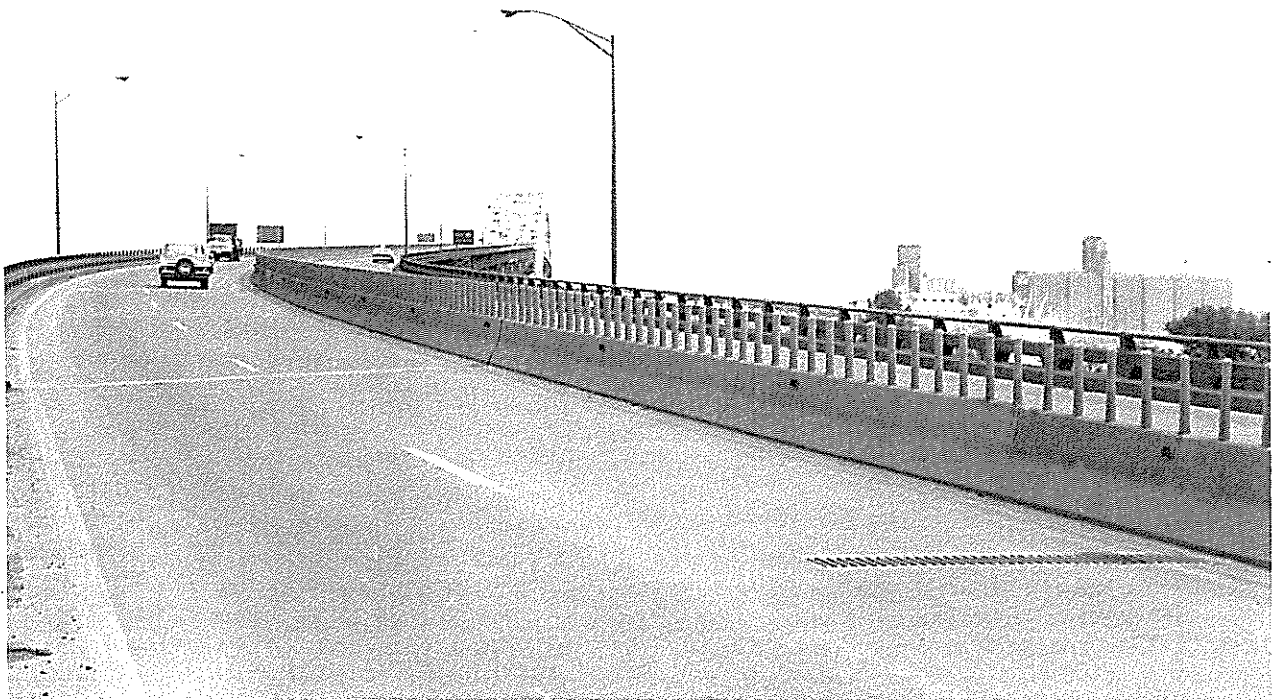
Figure 6. Paddles (type III) used as screen block opposing headlights at predetermined angles but permit surveillance of and access to the opposing lane by police and emergency personnel.
