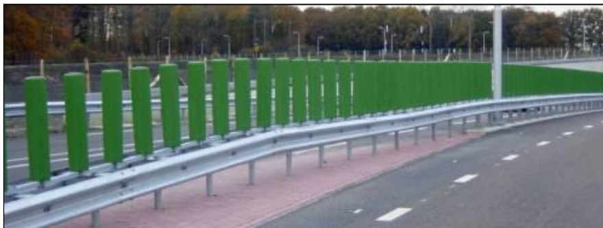
Figure 2.19: Beilharz Anti-Glare Screen System Source: (Beilharz Road Delineation Systems 2013)
