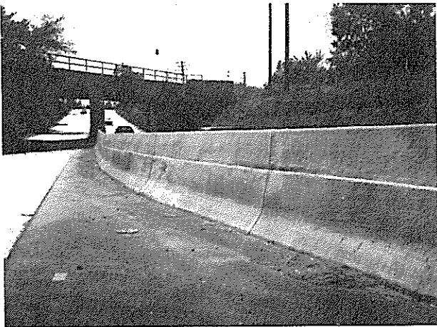
Figure 2. Type I glare screen is effective in eliminating glare sources from both wide and narrow angles.
