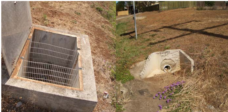
Figure 5-1 Current overflow structure and outlet
