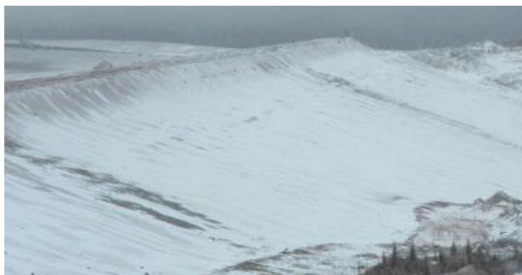
Figure 3.4: Large tailings embankment dam in Fermont, Quebec
