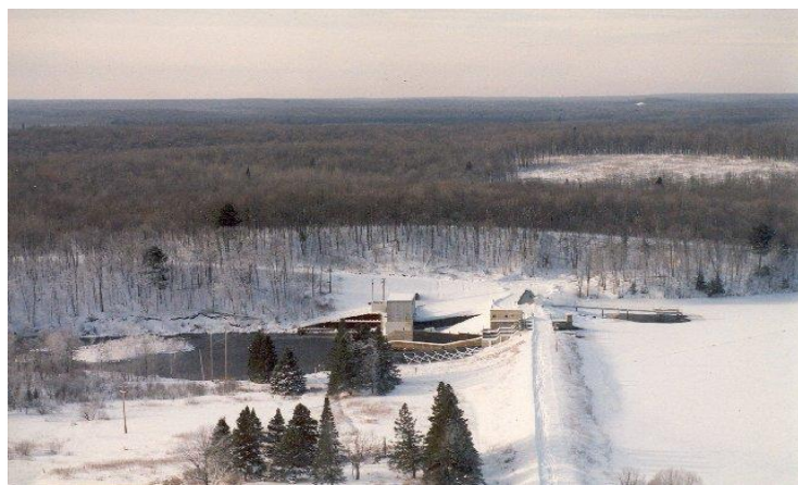
Figure 1.5: Chippewa dam and hydroelectric system during winter
