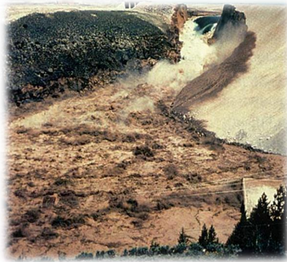
Figure 2.6: Failure of the Teton Dam in 1976 due to piping effects
