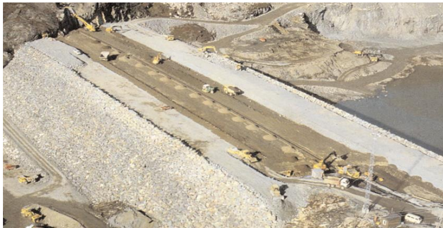
Figure 2.19: Construction of an Asphalt Core dam in Norway
