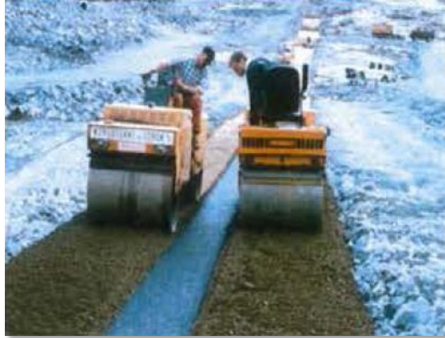
Figure 2.18: Compaction of asphalt concrete (AC) core and filters in AC core rock-fill dam (Høeg 1993)
