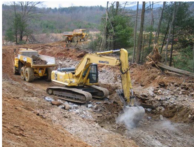
Figure 2.15: Removal of weathered rock during foundation preparation work (USBR 1984)
