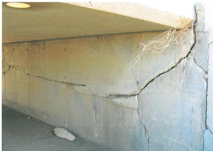
Figure 2 - Image of damaged abutment wall of culvert at East Warianna Creek
